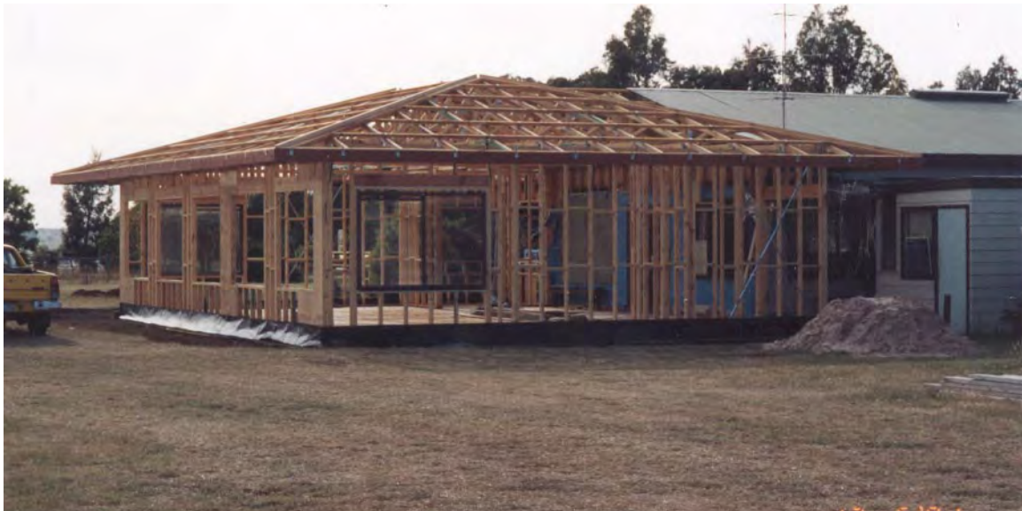
Above: Building of Clubhouse Extensions
