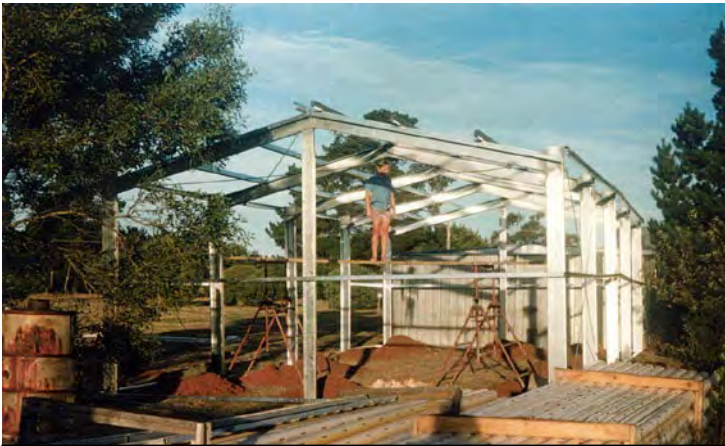
Above: Construction of Machinery Shed.
